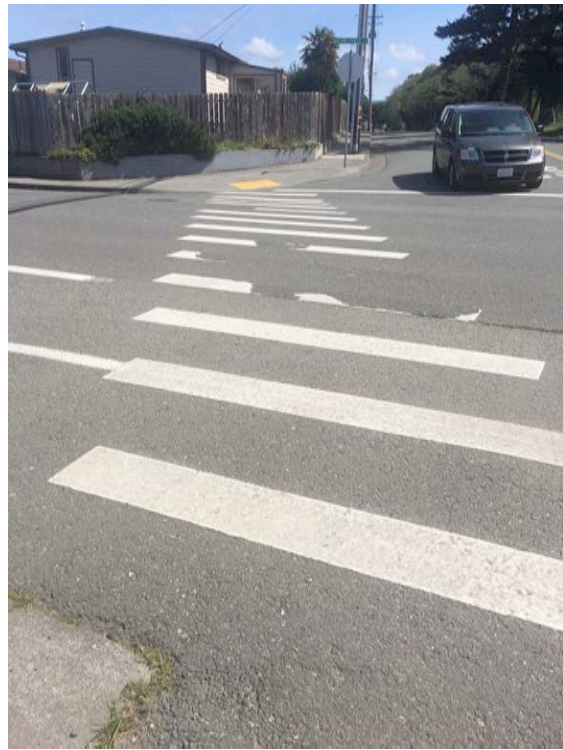
Figure 15: Crosswalk at McKinleyville Ave. & Railroad Dr. is faded.
