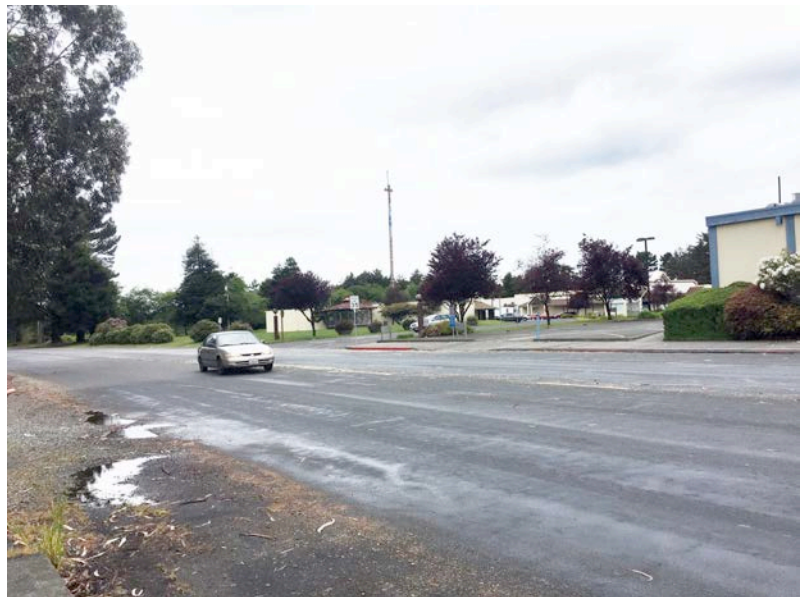
Figure 6: Lack of crosswalks across driveways leading from Hiller into shopping center
