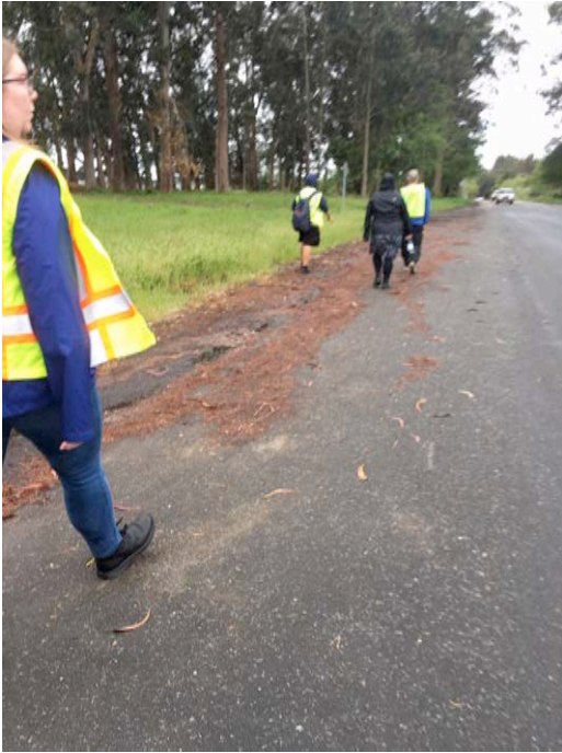
Figure 7: Inconsistent striping and lack of sidewalks and pedestrian lighting on Hiller Ave.
