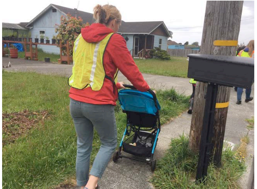
Figures 12 & 13: Many utility poles obstructing sidewalks on McKinleyville Ave.
