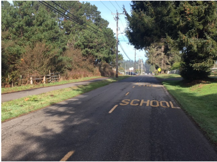
Low cost asphalt path along rural Dows Prairie Road.
