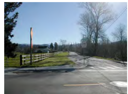
The corridor parallels Chartin Road in Blue Lake, where recently constructed sidewalks and curbs are paved over the A&M corridor.
