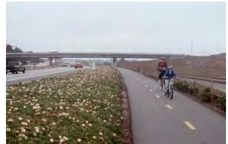
This multi-use trail and State Route 101 north of Monterey are separated by landscaping.
