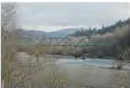
The steel truss A&M bridge spans 505 feet across the Mad River.
