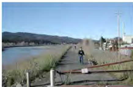
The Blue Lake Business Park Loop Trail is under development – this portion on the levee is in use.
