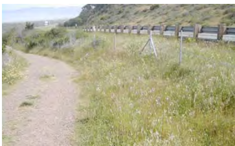
This relatively new segment of the Hammond Trail was surfaced with crushed shale.
