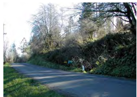
This road cutbank above West End Road would be moved back about 20 feet to move West End Road south and provide more space for a trail and driveway.
