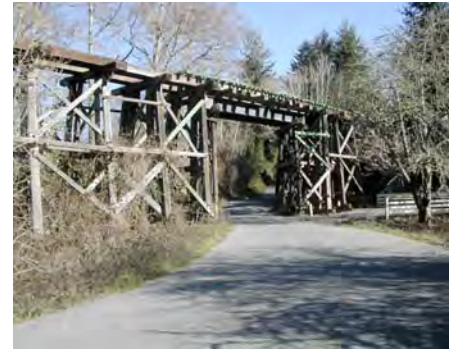
The Warren Creek Trestle spans Warren Creek Road.
