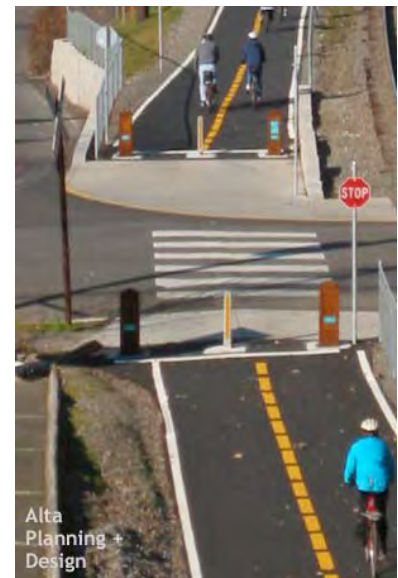
This Portland, Oregon rail-trail road crossing uses signage and striping to alert trail users and motorists.
