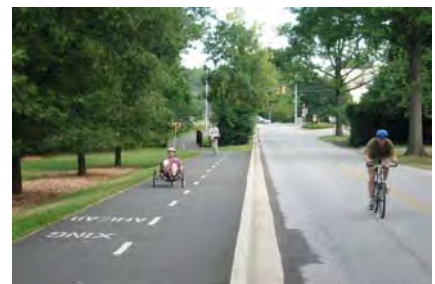
Separation of this rail-trail and roadway are achieved by a curb.
