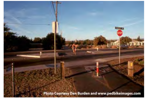
This trail/road intersection includes a median refuge, bollards and trail stop signs.
