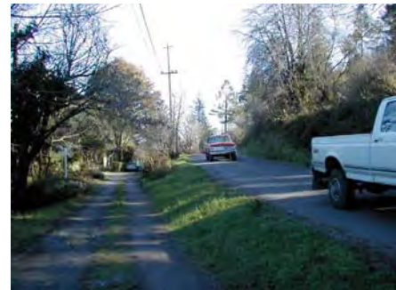
The A&M corridor and West End Road are too close to fit a trail between them without reconfiguration.
