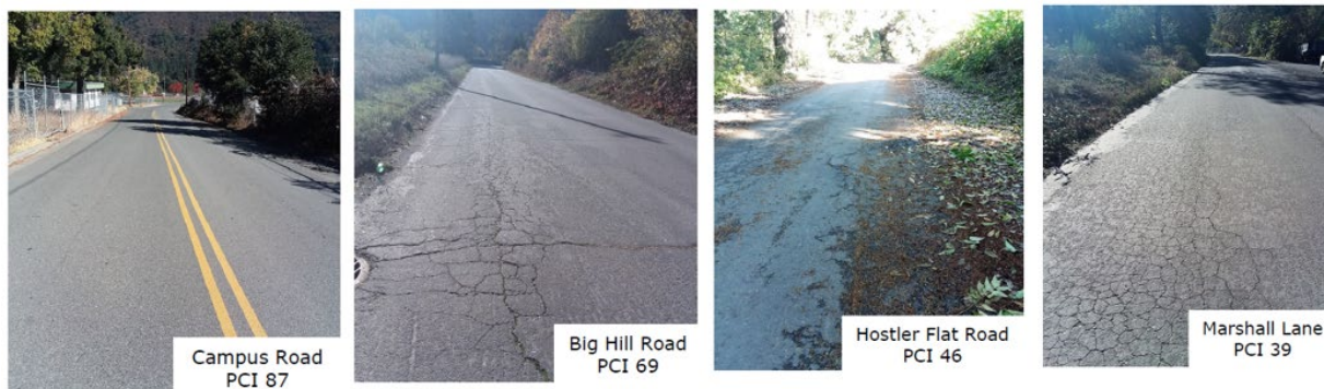
Figure 2. Examples of Roadways with Different PCIs Maintained by Hoopa Valley Tribe
