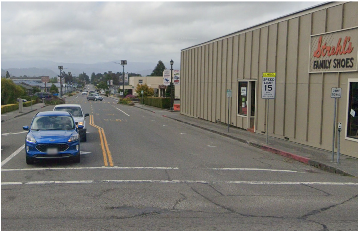
Figure 2.1 School Zone Speed Limit Sign on 12 th Street
