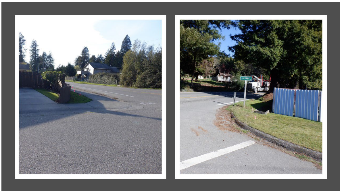
Figure 18. Site Walk Images Taken From the Stop Bar on Acacia Drive Facing Blue Lake Boulevard to the West (Left) and East (Right). Impaired Sight Distance was Observed in Both Directions.
