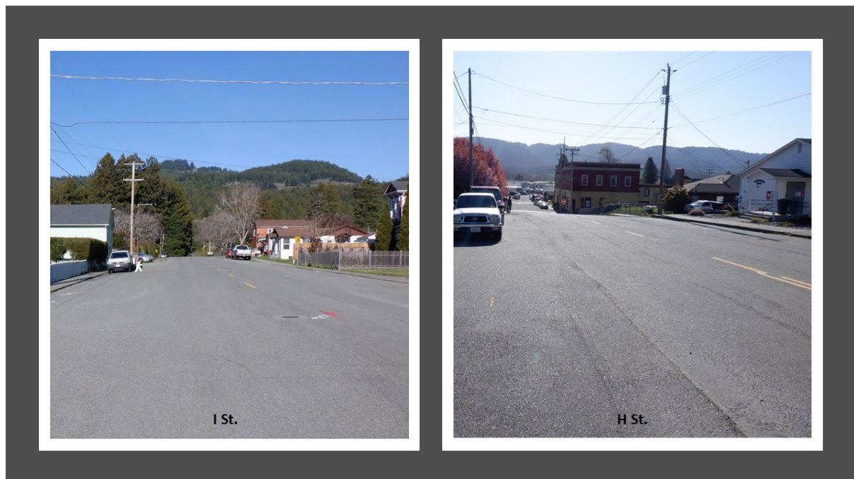
Figure 19. Site Walk Images Taken at the Crosswalks on "I" (Left) and H (Right) Streets. Potential risk factors were noted including wide lanes, the presence of on-street parking, and issues related to pedestrian crossing such as crossing distance and a lack of warning signage.
