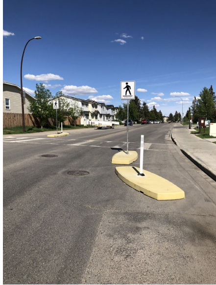
(Temporary Traffic Calming Curbs, Calgary, AB)
