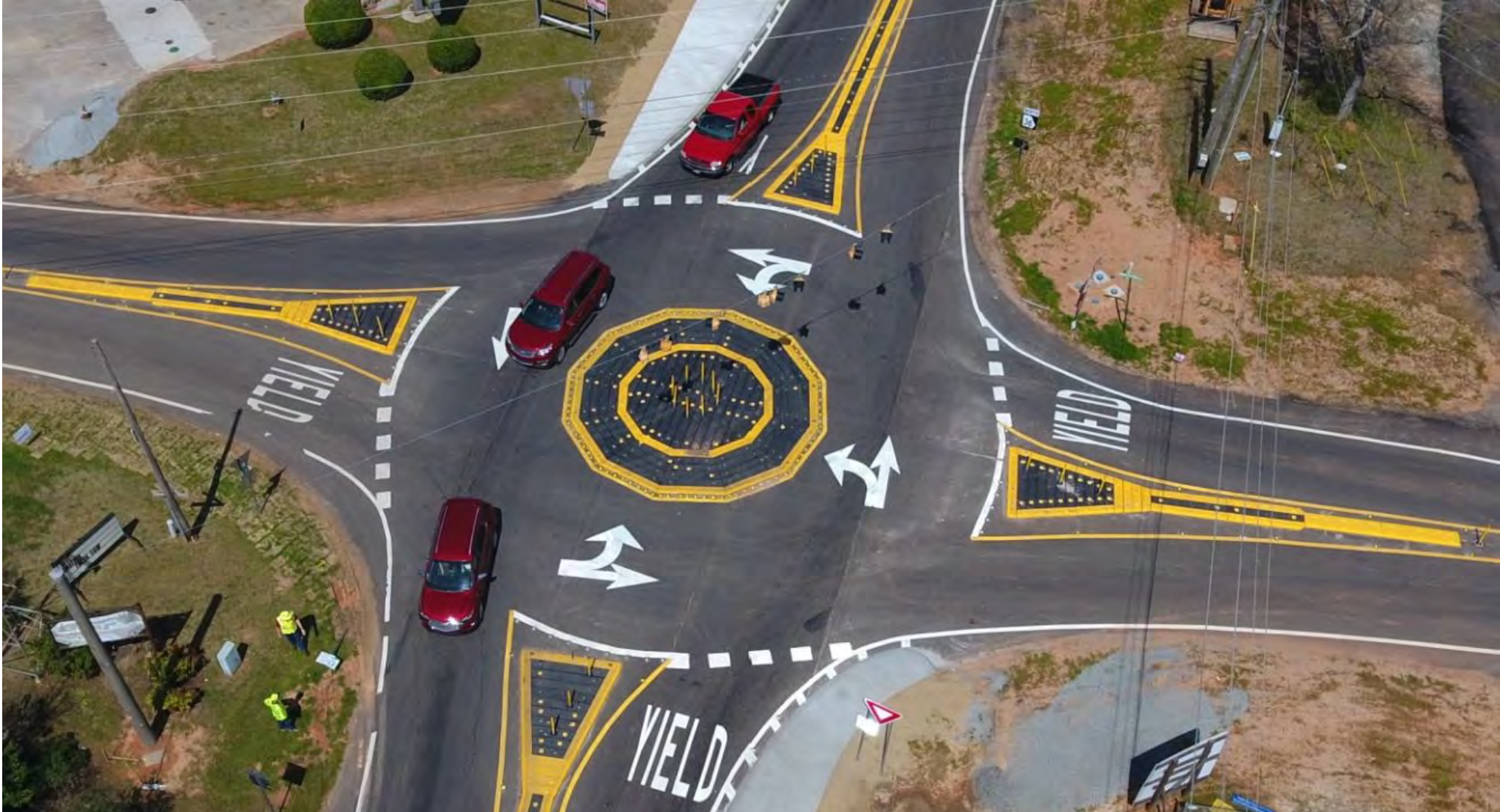
Example of quick-build and mountable small roundabout.
