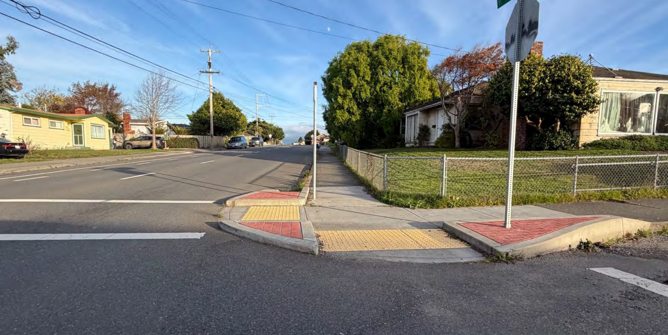
Example of new curb extensions in Eureka.
