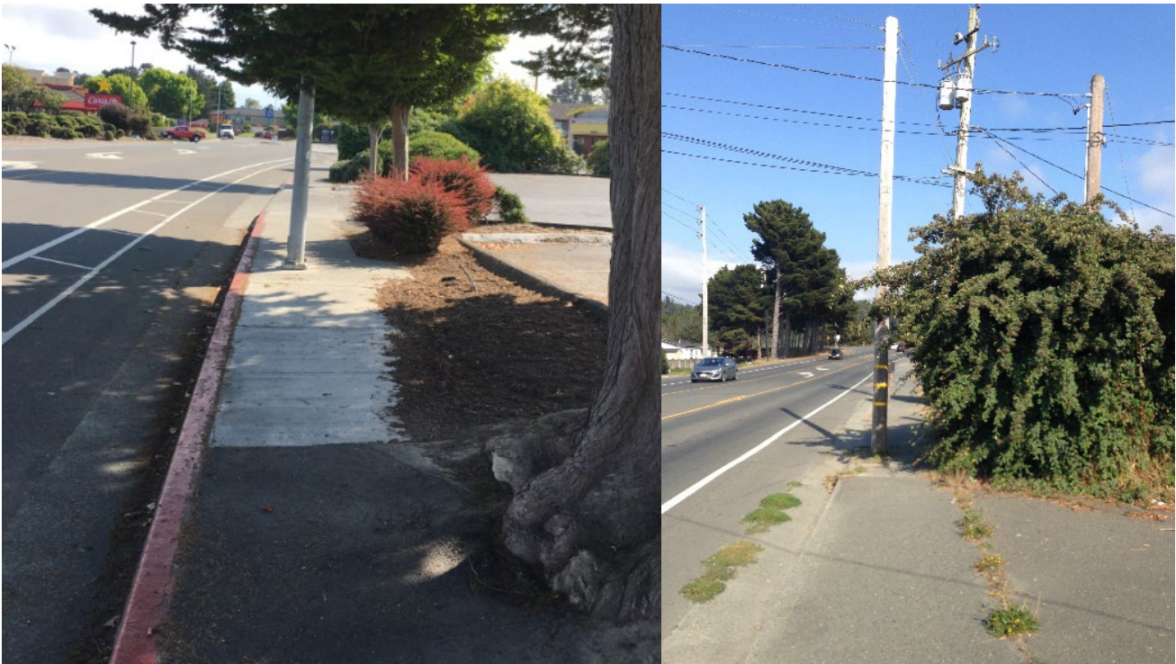
Narrow sidewalk with light post and overgrown tree roots creating barriers for pedestrians along Valley West Boulevard (left). Overgrown shrubbery limits walkability along Valley East Boulevard (right).
