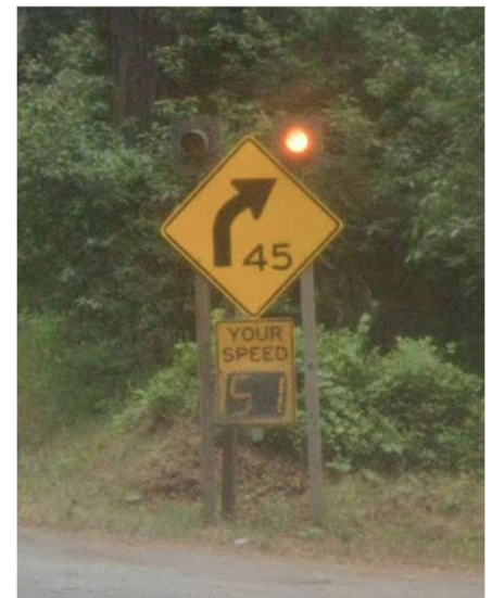
Figure 3.1 Dynamic / Variable Speed Warning Signage
