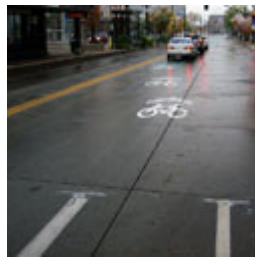
To transition bicyclists across traffic lanes or from conventional bike lanes or cycle tracks to a shared lane environment.
