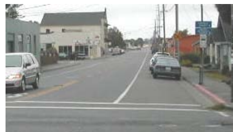
Fog lines striped on 11th Street in Arcata
