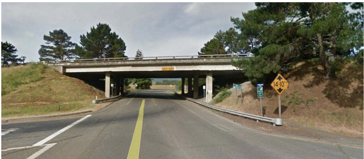
Figure 5: View of Kenmar Road Undercrossing
