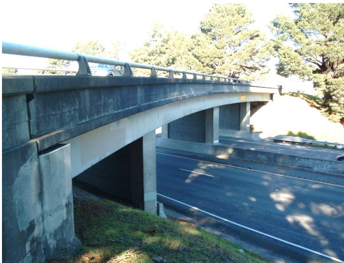
Figure 29: 12th Street Overcrossing - Looking East
