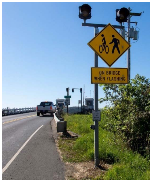
Figure 51: Example Activated Warning Signage Indicating Bikes on Bridge
