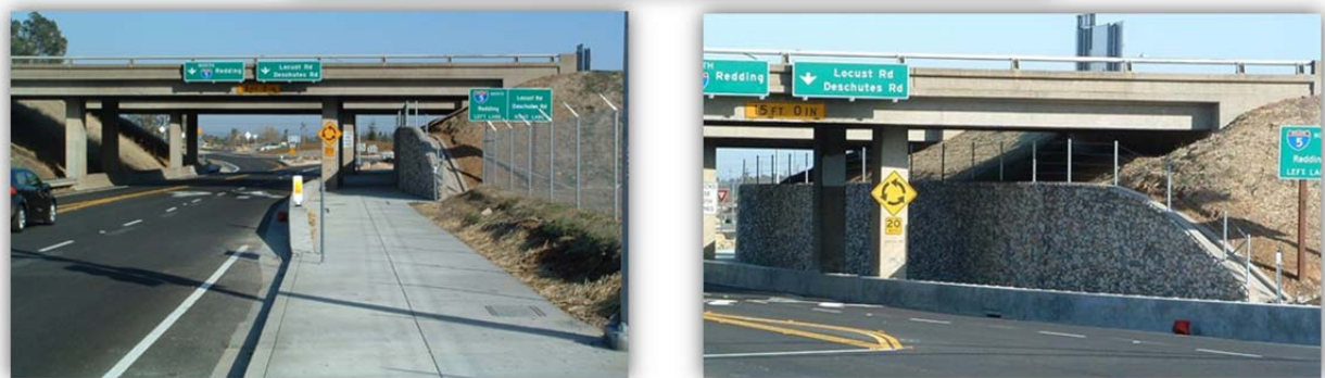
Figure 25: Example of path behind existing structure columns
