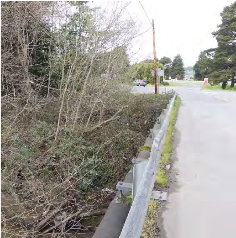
Riverwalk Drive bridge, looking east toward Hwy 101
